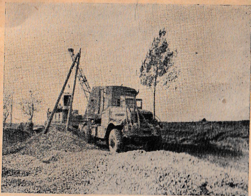
Loading gravel at Parroy, France.
