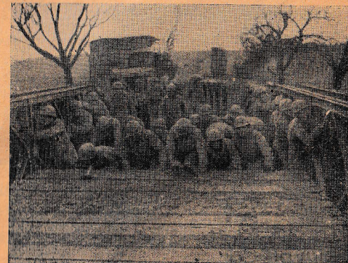
Pushing out Bridge at Woelfling, France.
