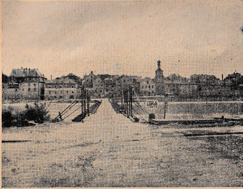
Fred K. Lawson Memorial Bridge on Danube at Regensburg, Germany.
