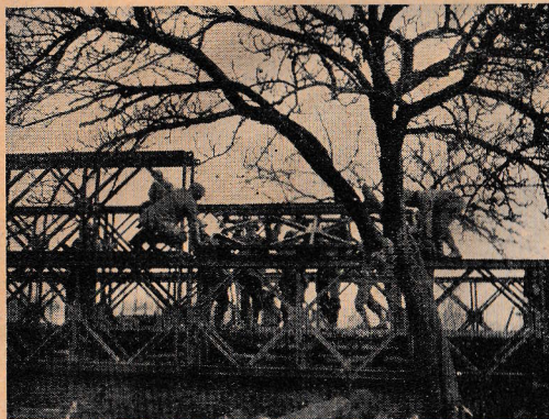
Construction of Bailey Bridge at Neufuallage, France.
